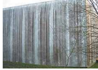
Above left: Wall covered with fungal growth ( Alternaria sp.).
