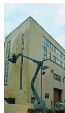
Building before and after cleaning with AlgoClear
